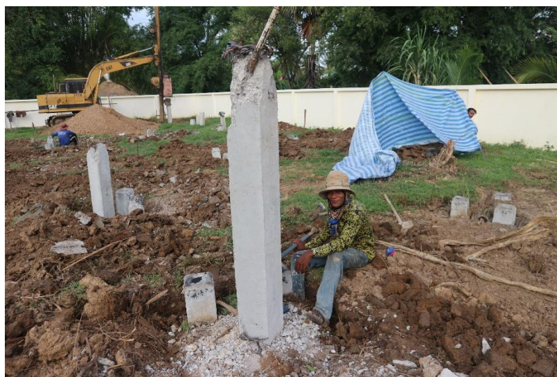
Foundations of the new building
